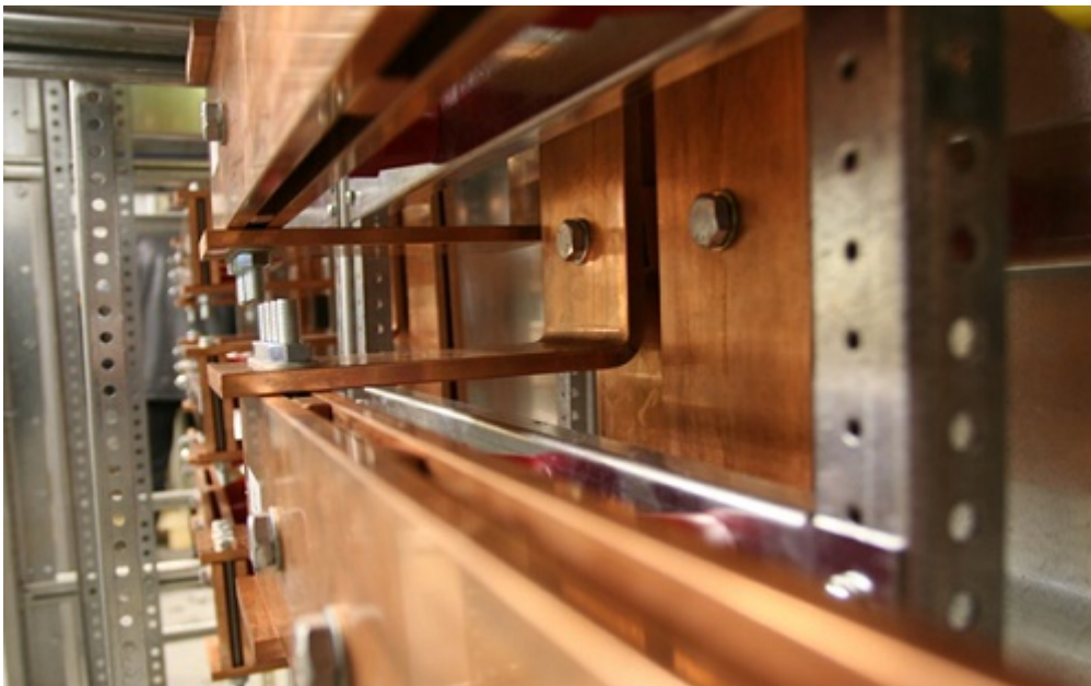
Figure 1 - Busbars system [1]
