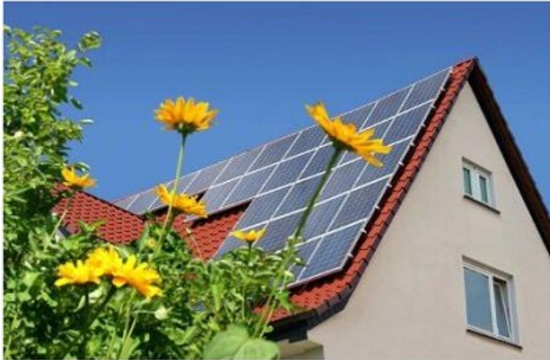
Figure 2 - Solar Panels used as source of energy in home
