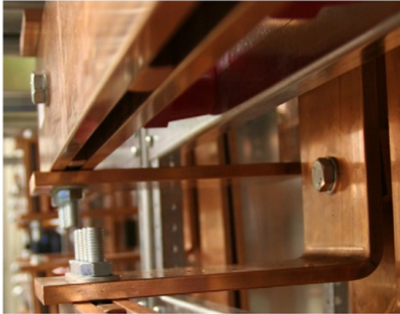
Figure 3 - Installed busbar
